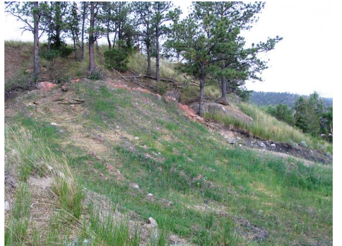
Republic No. 4 (coal), June 2006 photo: recent reclamation to close mine adit
