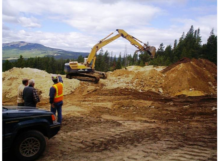
Ontario Mine August 2005 photo: excavation of approx. 10,000 cu. yd. of waste material contaminated with arsenic, barium and lead
