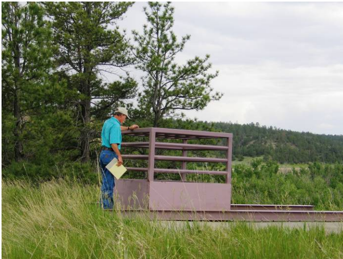
Republic No. 4 (coal), June 2006 photo: bat cupola erected with closure of vertical opening
