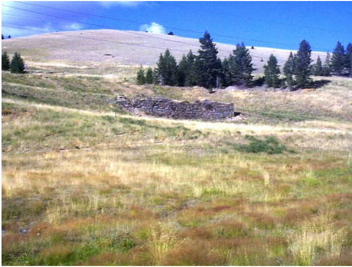
Gregory Mine (hardrock mine, mill & smelter), August 2005 photo: 91,000 cu. yd. of mine waste removed & transported to repositories; rock foundation left as evidence of historic mining
