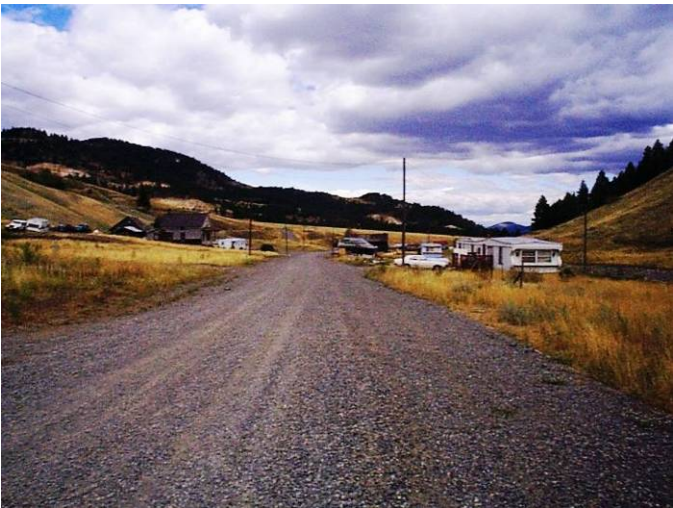
Wickes community August 2005 photo: after removal of 104,000 cu. yd. of heavy metal contaminated smelter wastes from residential areas, demolition & removal of two hazardous smelter stacks
